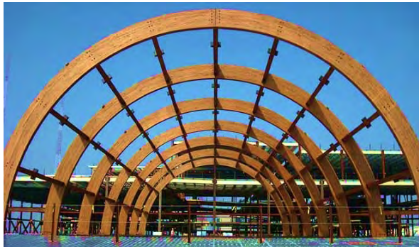
Atrium Roof for Meadowlands Xanadu in East Rutherford, NJ
